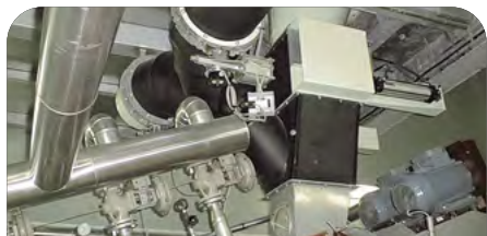
Screw - conditioner connection
